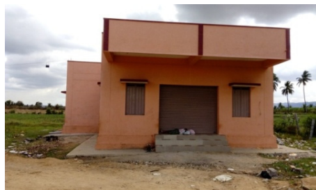
Dormitory at Galiyamma temple in Hosapete taluk remaining unused
